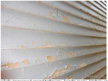
into the siding and wets the paint. The problem is particularly pronounced around bathrooms, laundry rooms, kitchens and other areas of high humidity. To reduce water vapor in the house, vent high humidity areas such as kitchens and bath areas to the outside. Clothes dryers should be vented directly to the outside and not to the attic, basement or crawl space. Mechanical humidifiers add large quantities of moisture to the air and should not be used if paint peeling is a problem.
