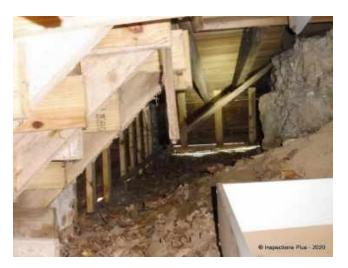
• **Repair:** Wood soil contact at the front porch structure should be eliminated wherever possible. This condition risks additional rot and insect activity.
