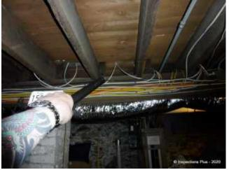
Some older homes have plaster ceilings in the basement. This material performs the same fire blocking function. However plaster has a life of about 50-75 years and is often deteriorated or has been penetrated to allow the trades to run their wires, pipes, and other mechanical penetrating items.
