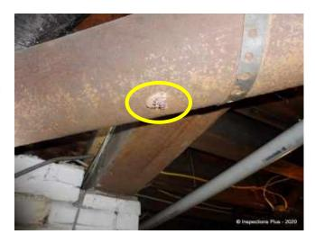
Some professionals and homeowners only patch the areas showing external signs of failure. This method is temporary since the failure of the cast iron pipe is already underway but may not yet show the external signs in the thicker walled areas. A permanent repair is replacement of all the cast iron, usually by white PVC pipe. Consult a licensed plumber.
