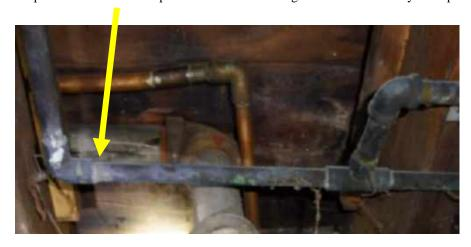
• Major Concern, Further Investigate, Repair: The cast iron waste piping is very old, fully depreciated, beyond its useful life and prone to unexpected leaking. Since this type of piping corrodes uniformly from the inside out, replacement of more than one section at a time may be required. This repair can become expensive if many sections of pipe are involved.
