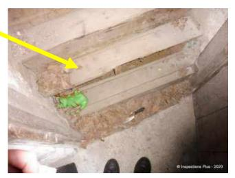
• **Improve:** Some fire-blocks in this house have been altered, damaged or removed. Fire-blocks slow down the progress of a fire giving your family a better chance to escape and the fire department a better chance of saving the house. They work by blocking the free flow of air. In general, very old houses used concrete, plaster and bricks, older homes use solid wood and newer homes use "fire-stopping" sealants approved for use by the local building code.
