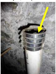
piping in the basement should be corrected. Although the open cast iron pipes in the basement are for abandoned downspout connections (from the outside), the pipes still connect to the active sewer connection which can let sewerage, and sewer gases into the home. Consider removal and appropriate termination of this abandoned piping.
