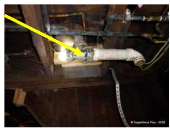
• **Further Investigate, Repair:** Upon review of pictures taken in the 3<sup>rd</sup> floor bathroom, the right side sink waste piping does not appear to be properly vented. The vent pipe appears to terminate inside the cabinet, behind the sink. A licensed plumber should be engaged to further investigate. Repair can become complicated if the sink(s) in this bathroom
